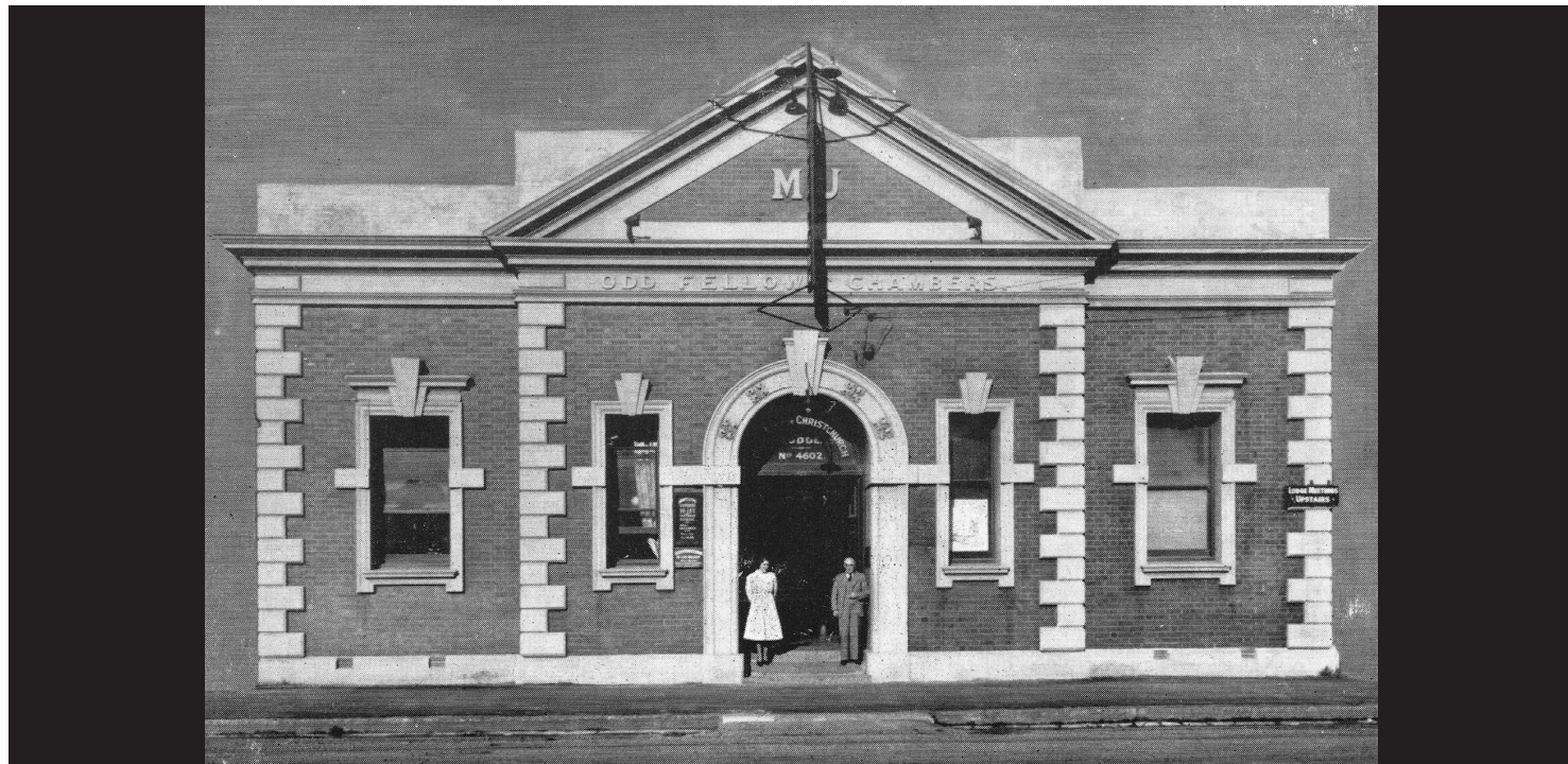
The Manchester Unity Lodge Hall, circa 1904 (photo courtesy of Archives at the Ferrymead Heritage Park).
