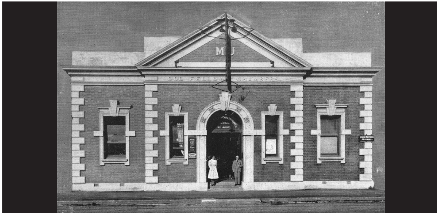
The Manchester Unity Lodge Hall, circa 1904 (photo courtesy of Archives at the Ferrymead Heritage Park).
